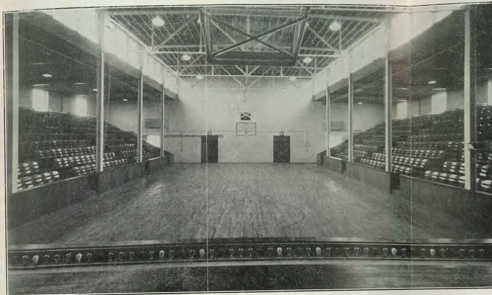
INTERIOR VIEW JASPER HIGH SCHOOL GYMNASIUM
